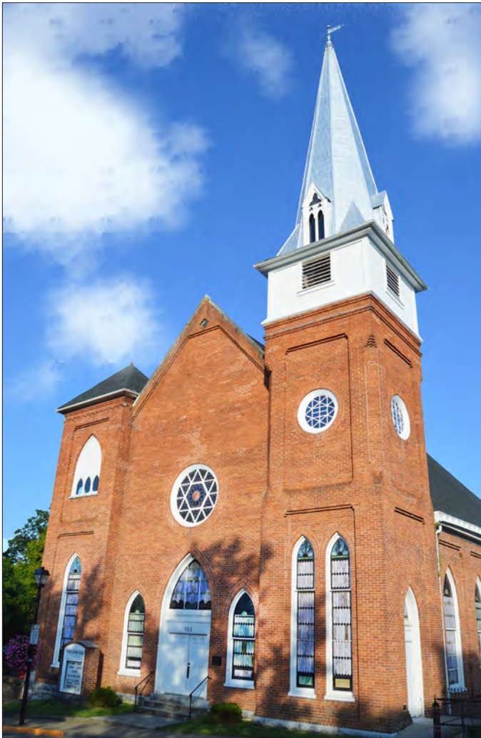
First Baptist Church of Lexington, built by its members, 1894–95, and now on the National Register of Historic Places
